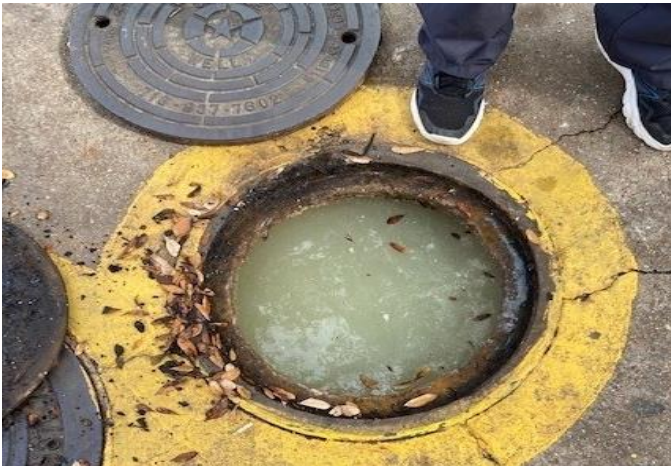
Sewer backup in COH manhole on Morningside Dr.
